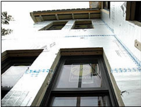
A superinsulated home with foam insulation placed on the outside of the walls and on top of the existing roof. (Martin LaMonica/CNET Networks)
